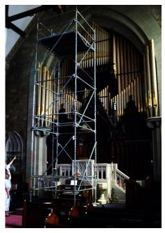
It looks as though a cage has been built to keep the organist from getting away, doesn't it? Well, it's actually scaffolding that was assembled on the chancel and in each balcony in order to replace the fire sensors way up in the ceiling. The equipment has been installed and the scaffolding is gone now. Meanwhile, the organ has had its annual tuning and maintenance and it is ready to liven up our hymn singing, as soon as it is safe to sing hymns again.
